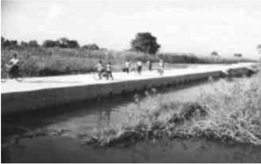
People crossing Sarju Nala after causeway construction
