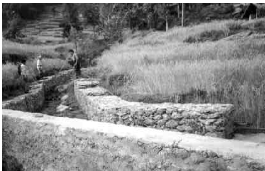
Check dam Construction, Sankhuwa-Sabha
