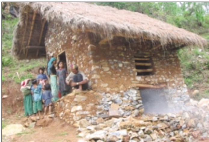
Pani Ghatta (Water Mill) construction support at Korchabang, Rolpa district
