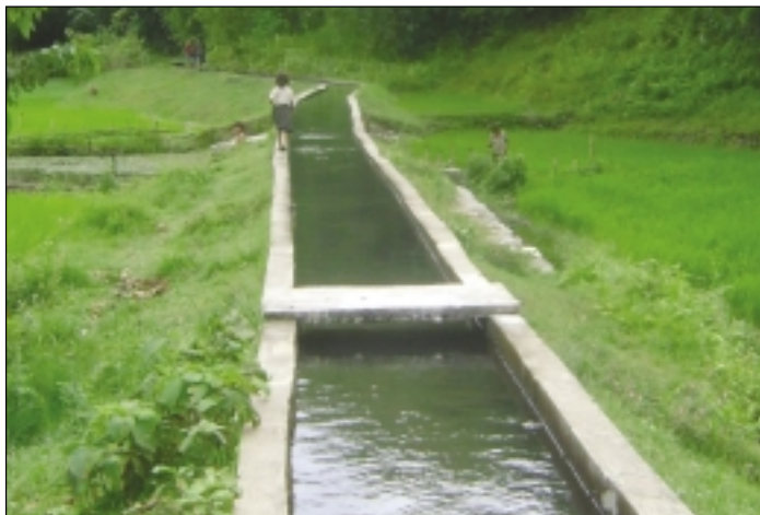
Irrigation canal built in Bayarban, Morang district
